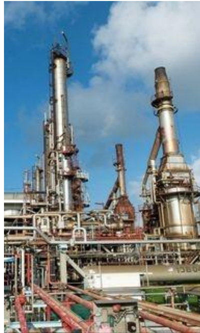
Renewable fuel oil for our industrial boilers
