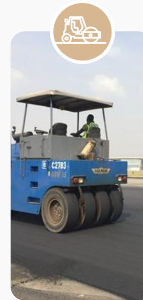
Road grades, modified bitumen, emulsions etc.
