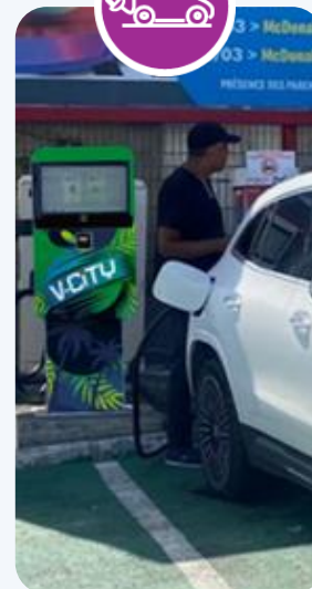
Charging stations, E-mobility solution
